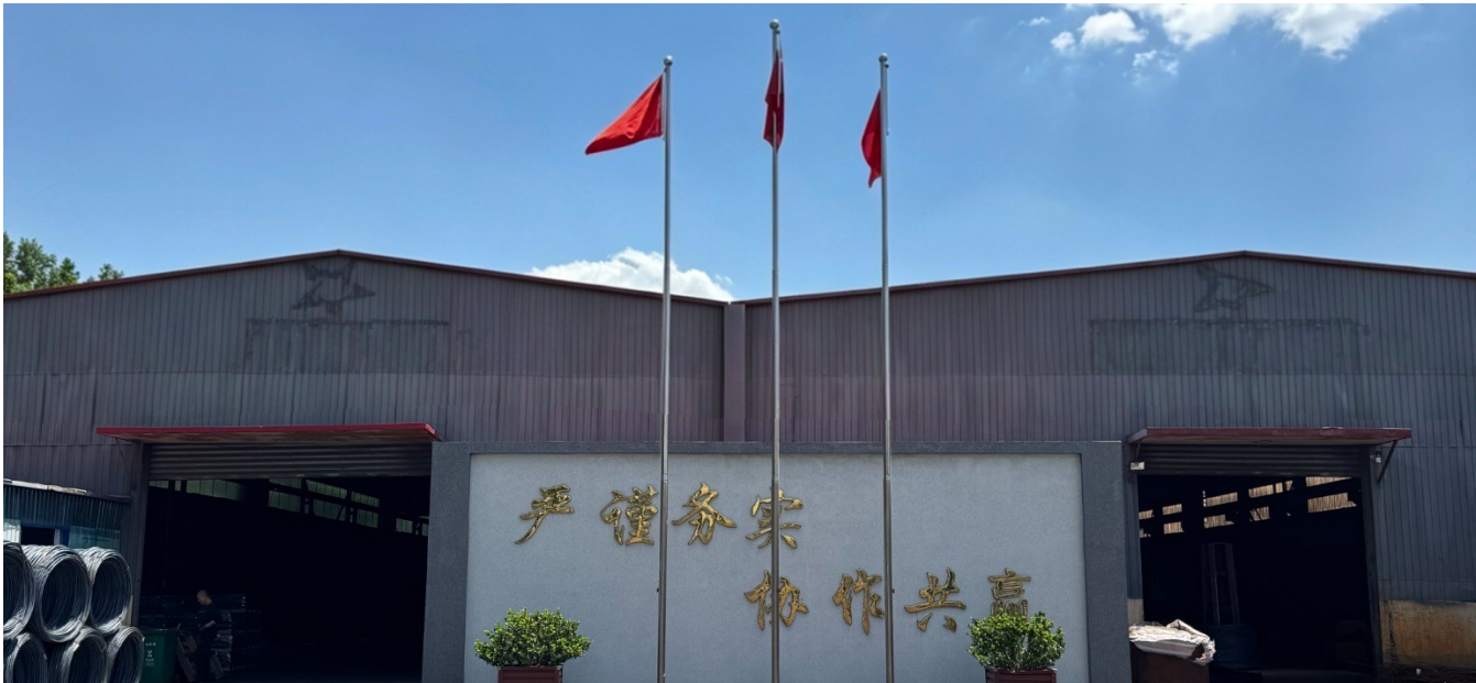
EVERSTAR MANUFACTURING SITE | WUJI, SHIJIAZHUANG, HEBEI, CHINA
