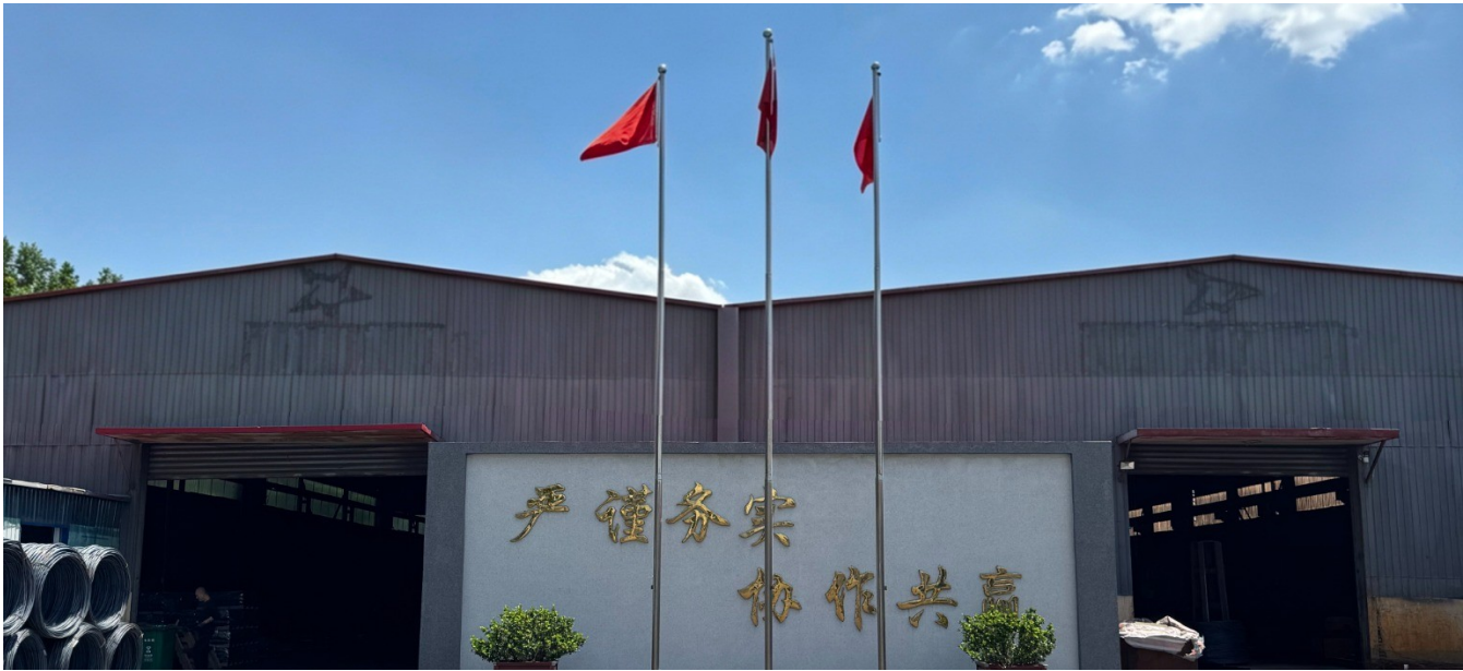
EVERSTAR MANUFACTURING SITE | WUJI, SHIJIAZHUANG, HEBEI, CHINA
