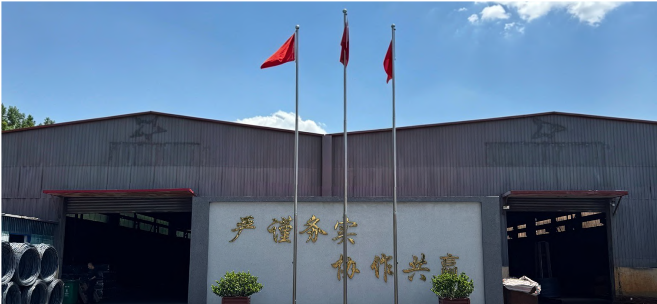
EVERSTAR MANUFACTURING SITE | WUJI, SHIJIAZHUANG, HEBEI, CHINA
