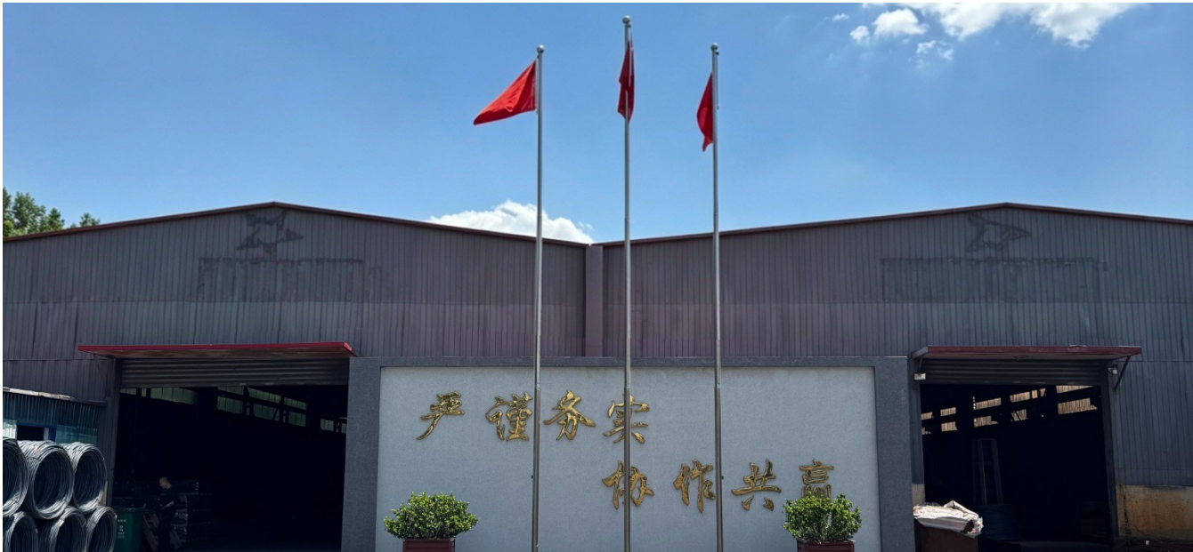
EVERSTAR MANUFACTURING SITE | WUJI, SHIJIAZHUANG, HEBEI, CHINA
